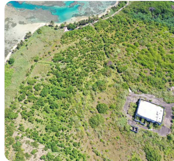
Through a successful methodology involving the construction of canals and direct mangrove planting, this military base in Galeta Island, Panama, has been restored into a thriving mangrove forest © Andrés E. Fraiz T., Wetlands International.
